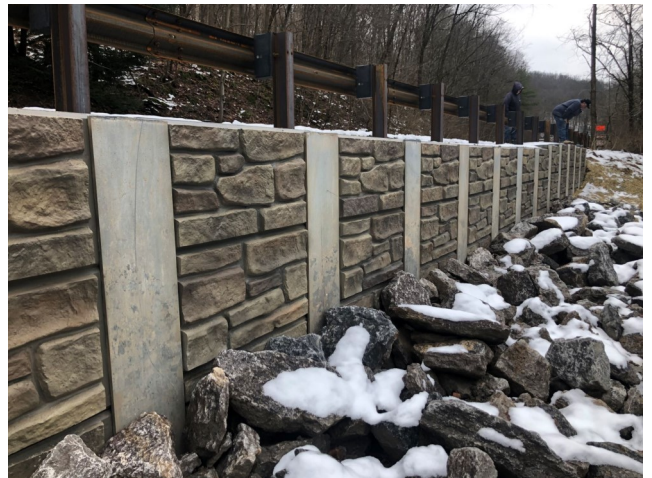
Soldier Pile Wall Construction Completed
