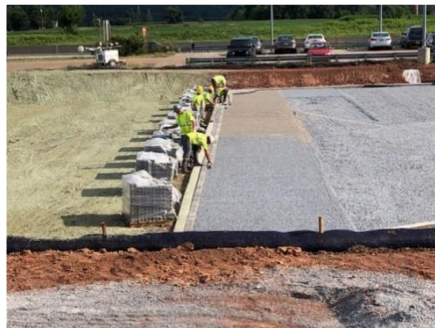
Placement of Pavers Begins
