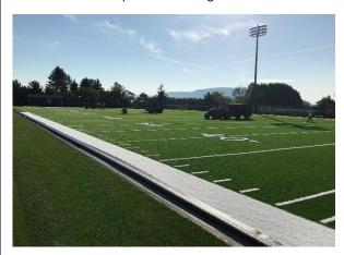
turf (approximately 190 feet by 390 feet) as well as the site design for a new trench drain, located on the western side of the field between the artificial turf surface and the grass field surface. Stahl Sheaffer finalized the design documents and prepared construction plans and technical bid specifications.
