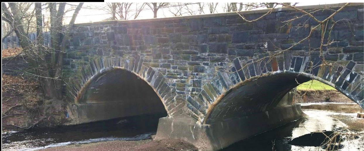
EXISTING STRUCTURE BEFORE CONSTRUCTION
