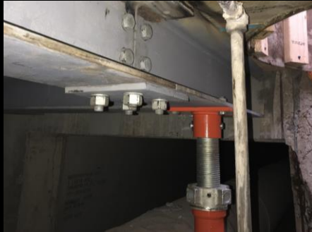
Construction Shoring & Falsework
