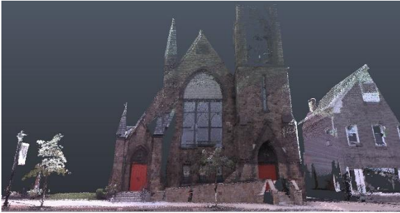
Fig. 1 – Point Cloud Image
